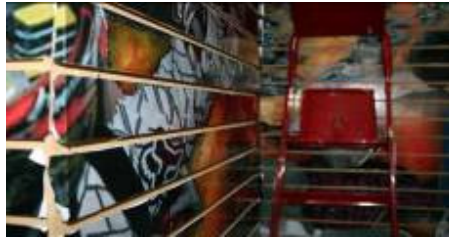
< Wood surface Failure>
